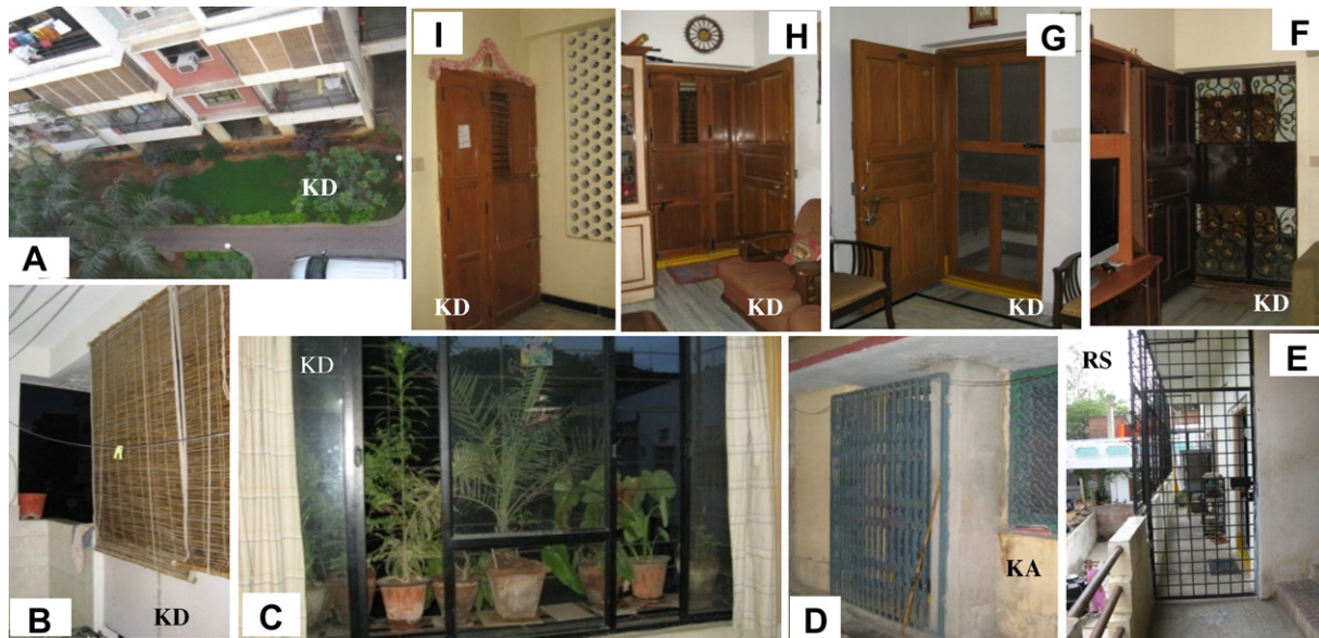
Fig. 10. Some adaptive interventions applied to windows, doors and balconies to promote higher adaptive use, as found in KD, KA and RS. (A, B): Bamboo blinds hung on balcony openings and (C) Planter box extension to windows to reduce glare and sunlight and curtains and to improve privacy, (D, E, F) : Metal grill gates to main doors and metal grill enclosures to balconies to improve safety, privacy and cross ventilation. (G) Additional door shutters with mosquito screens and vents for improved cross ventilation, (I) RCC Jalis applied to corridors for safety, sun control and cross ventilation.
